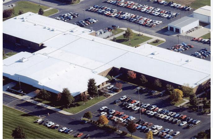
Other commercial roofing systems are prefabricated, like those made by Duro-Last Roofing, Inc. Because it's manufactured to precisely fit the specifications of your building, a Duro-Last roof eliminates most rooftop membrane seaming, greatly reducing the likelihood of installation errors and future leak problems.
