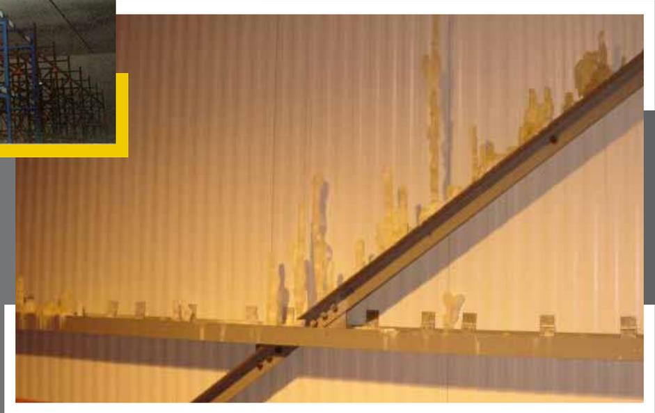
Moisture stored in the roof assembly will travel from one dew point location to another as the ambient outdoor temperature changes. In the summer, ice settles as the top melts and refreezes at a lower level. In the winter when the exterior temperature is cold, this moisture migrates up close to the underside of the membrane, condenses, and returns to the lower levels during the next warm cycle.
